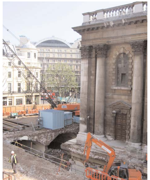
The excavation and demolition around the church progresses
