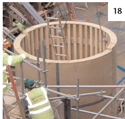
to house the Connection at St Martin's during building work is brought on site and assembled (18) A wooden template for the new lift is constructed.
